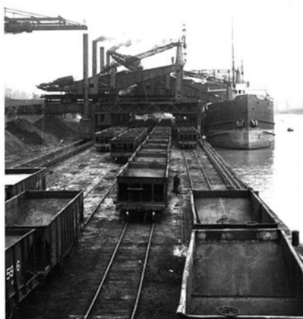
Despite its drawbacks, the Hulett proved its worth. It could dig 17 tons of ore from a vessel in fifty seconds. It was steam powered and did not require the expensive cables that other machines needed to operate.
